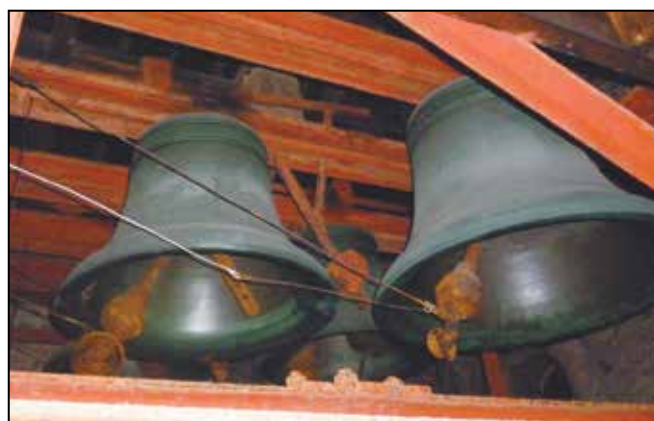
The bells held in their metal casing with clappers hanging and moved by wires
