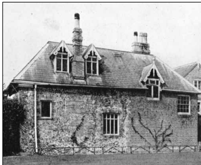
ABOVE: a view of the eastern wing as it was in 1950. The brick backing to a large fireplace can be seen in the centre of the old flint wall. There is modern brickwork to the far right.
