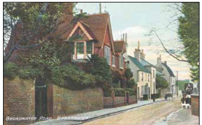
Two photographs of the original narrow street of Broadwater, before being widened in the 1930s and 1960s
