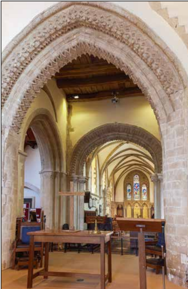
The rounded eastern Norman arch is framed by the pointed western arch
