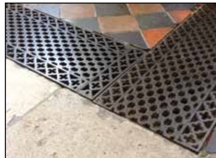
A length of the 1862 cast iron heating grille
