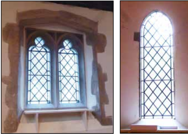
LEFT: Middle Ages-style ground floor aisle window RIGHT: lancet-style window at west end of each aisle
