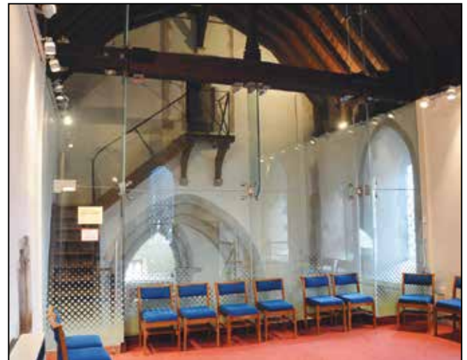
The glass screen of the mezzanine floor in the north transept
