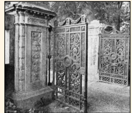
The western gates to the estate
